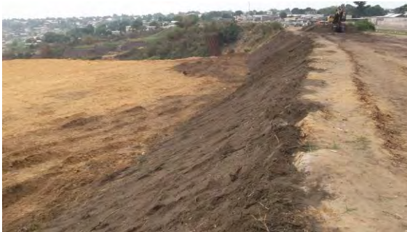
Photo 23. Mimi erosion site at Brazzaville before vetiver planting
