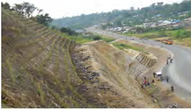
Photo 37. Planting vetiver on eroded slopes of road from Fortportal to Bundibugyo, Uganda Republic, august 2013
