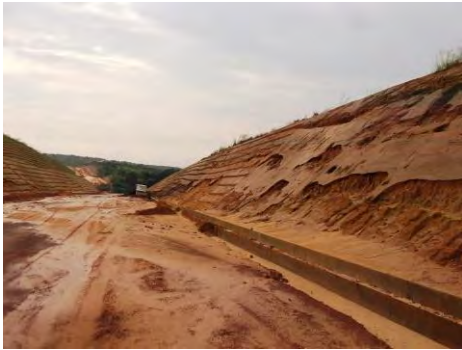
Photo 27: Water erosion on RN1 slope at Congo-Brazzaville
