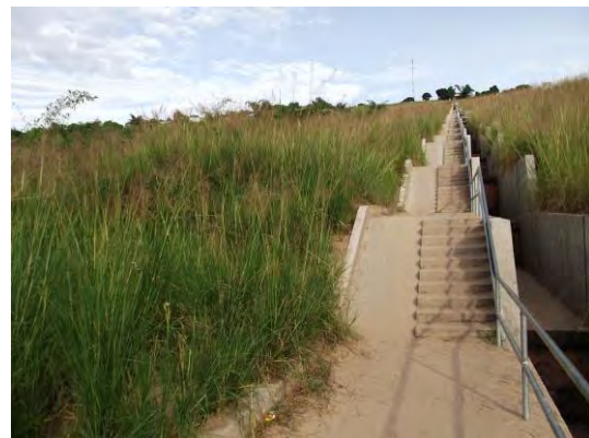
Photo 26. Pylône erosion site, 12 months later
