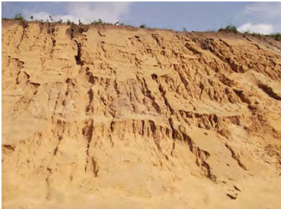
Photo 29. Eroded slope of Congo Brazzaville highway
