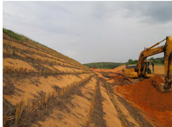
Photo 30. Planting vetiver on highway slope at Congo-Brazzaville
