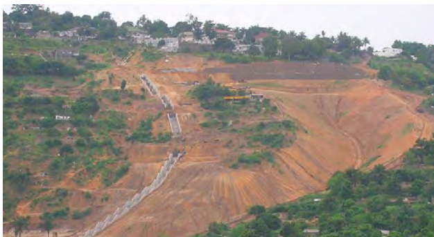
Photo 13. Drève de Selembao erosion control site before vetiver planting and hydroseeding
