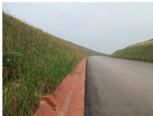
Photo 32. Congo-Brazzaville highway slope protected, 12 months after planting vetiver
