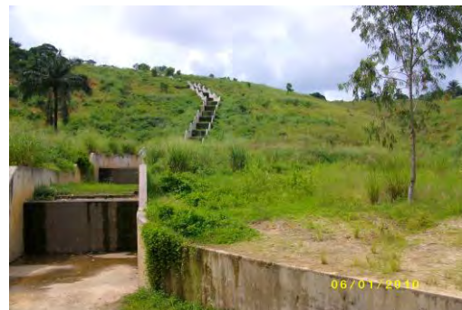
Photo 14. Same site 2 years later, after vetiver planting and hydroseeding
