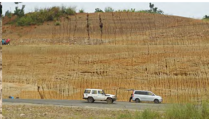
Photo 36 : Slopes erosion on road from Fortportal to Bundibugyo, Uganda Republic
