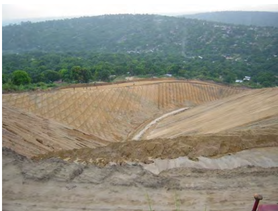
Photo 15. Drève de Selembao erosion control site before vetiver planting and hydroseeding
