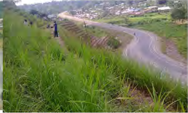
Photo 38. Slopes of road from Fortportal to Bundibugyo totally protected, 5 months later
