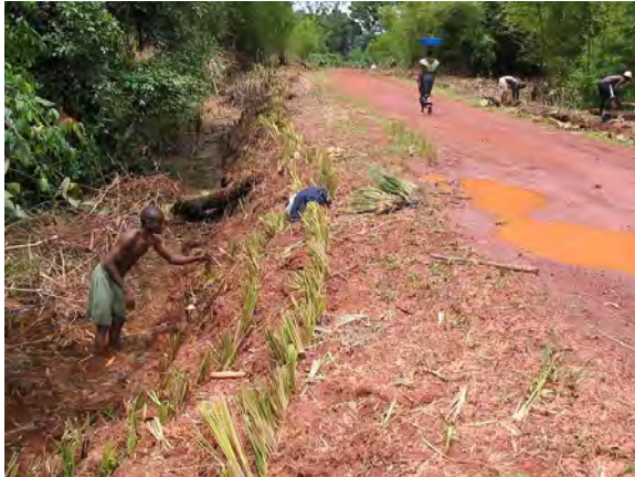
Photo 11. Planting vetiver for fill batter stabilization
