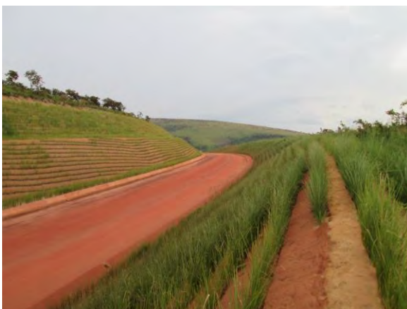
Photo 31. Congo-Brazzaville highway slope protected, 6 months after planting vetiver
