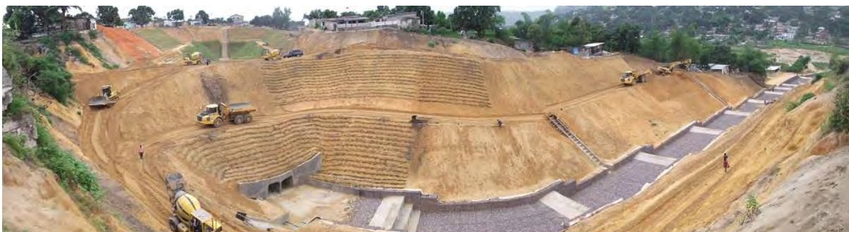
Photo 21. Vetiver planting on Boukeni erosion control site at Brazzaville
