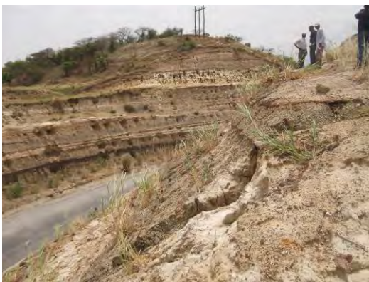
Photo 35. Slopes erosion on road from Fortportal to Bundibugyo, Uganda Republic
