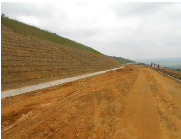
Photo 33. Planting vetiver on RN2 slope at Congo-Brazzaville
