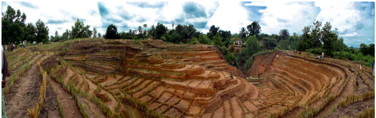
Photo 8. Panoramic site view after completed work
