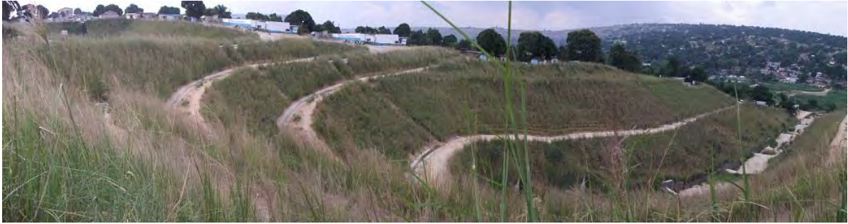
Photo 22. Boukeni erosion control site, 12 months after planting vetiver
