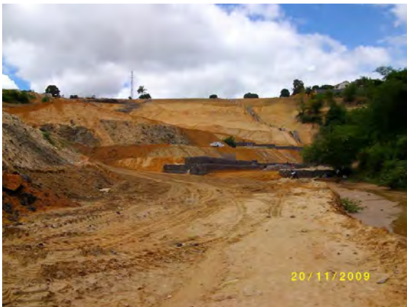
Photo 19. Casis erosion control site at Brazzaville, before vetiver planting
