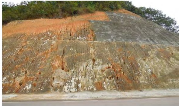
Photo 28 Water erosion on RN1 slope at Congo-Brazzaville
